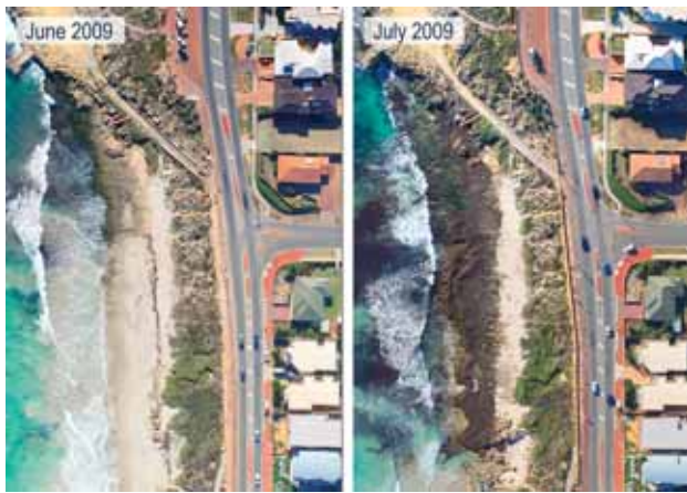
Aerial images showing erosion of North Beach in Perth after a winter storm.
