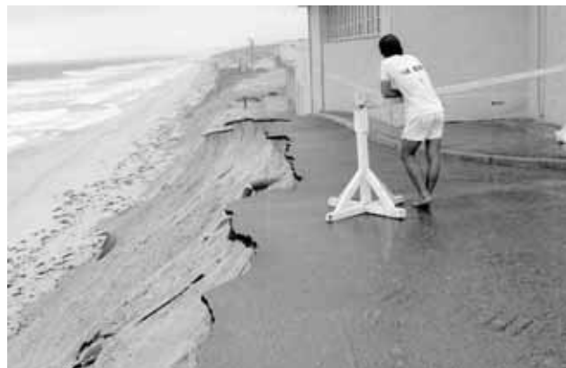
Erosion along Perth beach near Floreat Surf Club, 1978.
