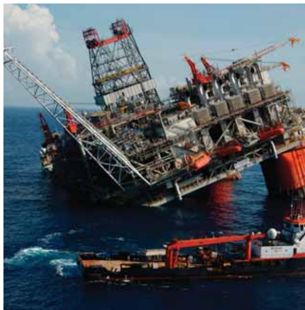
Hurricane-damaged oil rig Thunder Horse, in the Gulf of Mexico 2005, a semi-submersible platform owned by BP, was found listing after the crew returned. The rig was evacuated for Hurricane Dennis.
