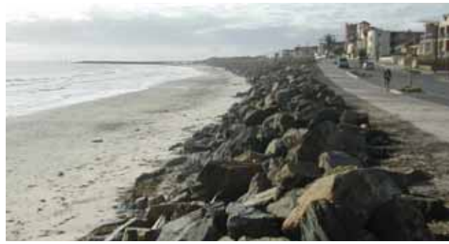
Rock seawall along Adelaide's West Beach.
