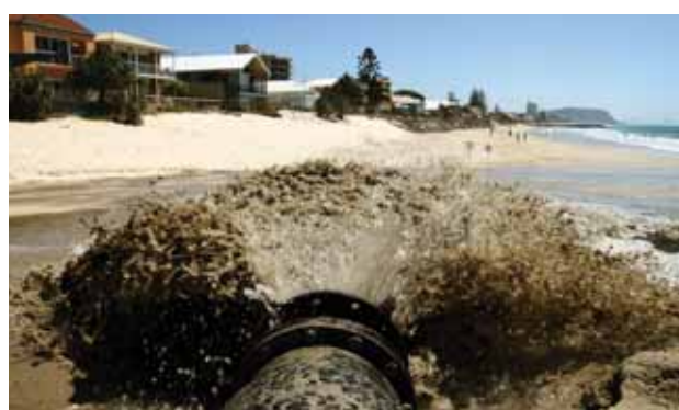
Sand pumping at Palm Beach, Queensland.
