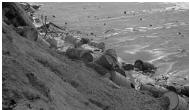
Forty-four gallon drums filled with concrete to prevent further beach erosion on the Gold Coast, 1967.
