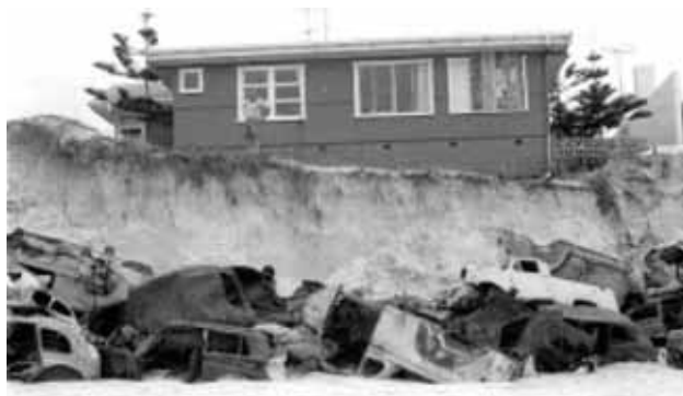
Car bodies used to try and stop the progress of erosion on the Gold Coast, 1967.
