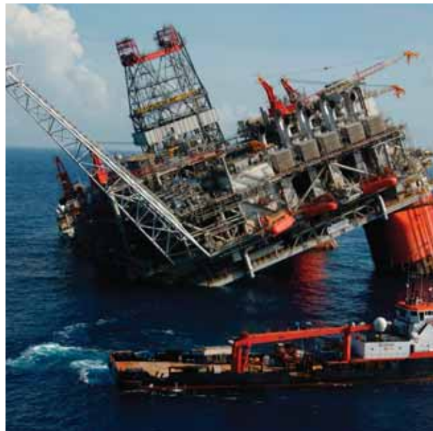
Hurricane-damaged oil rig Thunder Horse, in the Gulf of Mexico 2005, a semi-submersible platform owned by BP, was found listing after the crew returned. The rig was evacuated for Hurricane Dennis.
